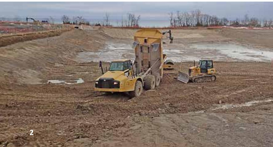
**Clean soil is delivered to remediated areas of the site along designated clean internal haul roads. Articulated rock trucks place the clean fill, in a controlled manner, for spreading and grading. Remediated areas of the site are separated by physical barriers from future excavation zones to prevent cross-contamination.**
