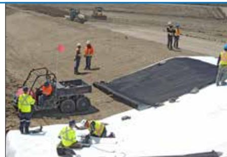
Installation of HDPE liner in Cell 1
