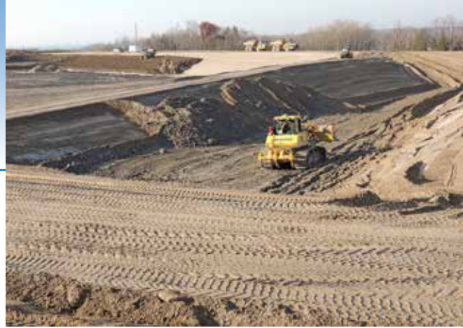
Cell 1 excavation in fall 2016
