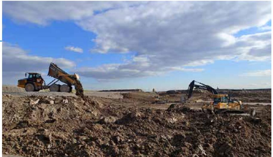
**Waste transported from the Lake Ontario shoreline site to the engineered facility is compacted to help form the future drumlin shape of the aboveground mound.**
