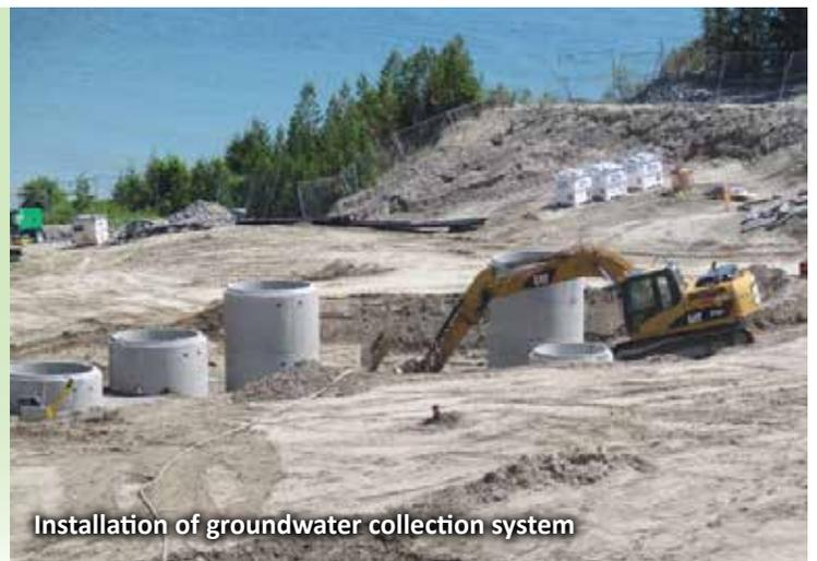
Installation of groundwater collection system
