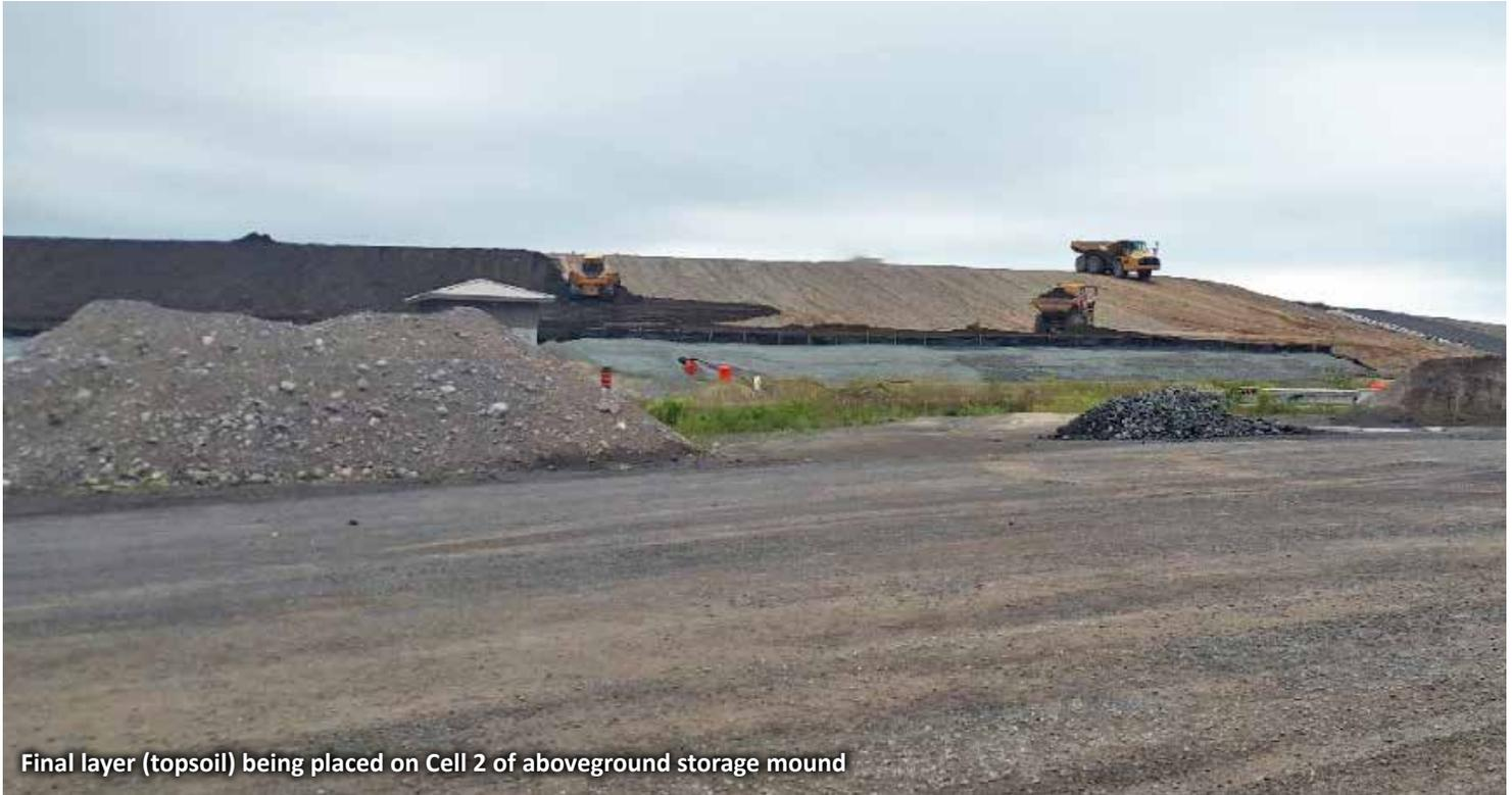
Final layer (topsoil) being placed on Cell 2 of aboveground storage mound
