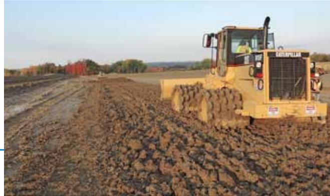
The mound's clay liner is being compacted by machinery known as a "sheep's foot roller."
