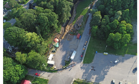
Strachan Street Ravine site restoration
