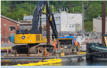
Port Hope Harbour remediation ongoing
