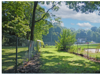
Lions Recreation Centre Park site preparation
