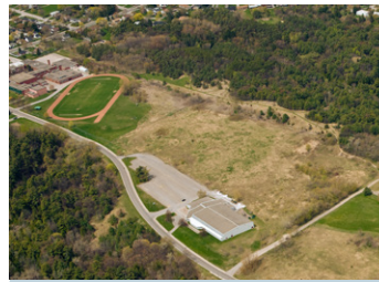
Highland Drive Landfill Area Site Prep
