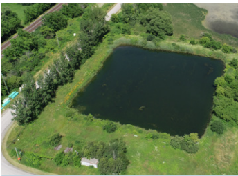
Chemetron Lagoon site preparation
