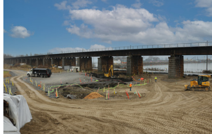
CN/CP Viaducts remediation underway
