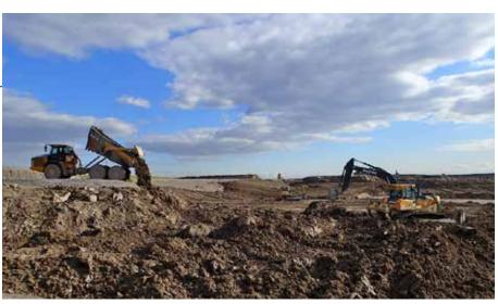
Waste transported from the Lake Ontario shoreline site to the engineered facility is compacted to help form the future drumlin shape of the aboveground mound.
