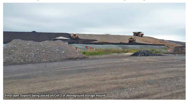
Capping and closing of the engineered storage mound at the Port Granby LTWMF is underway. The mound comprises two separate cells housing the low-level radioactive waste; each cell is being capped with multiple layers of natural and manufactured materials.
