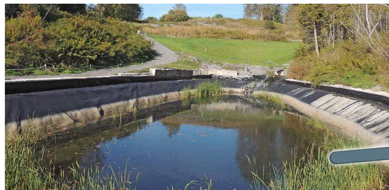
Existing waste water reservoirs and collection ponds
