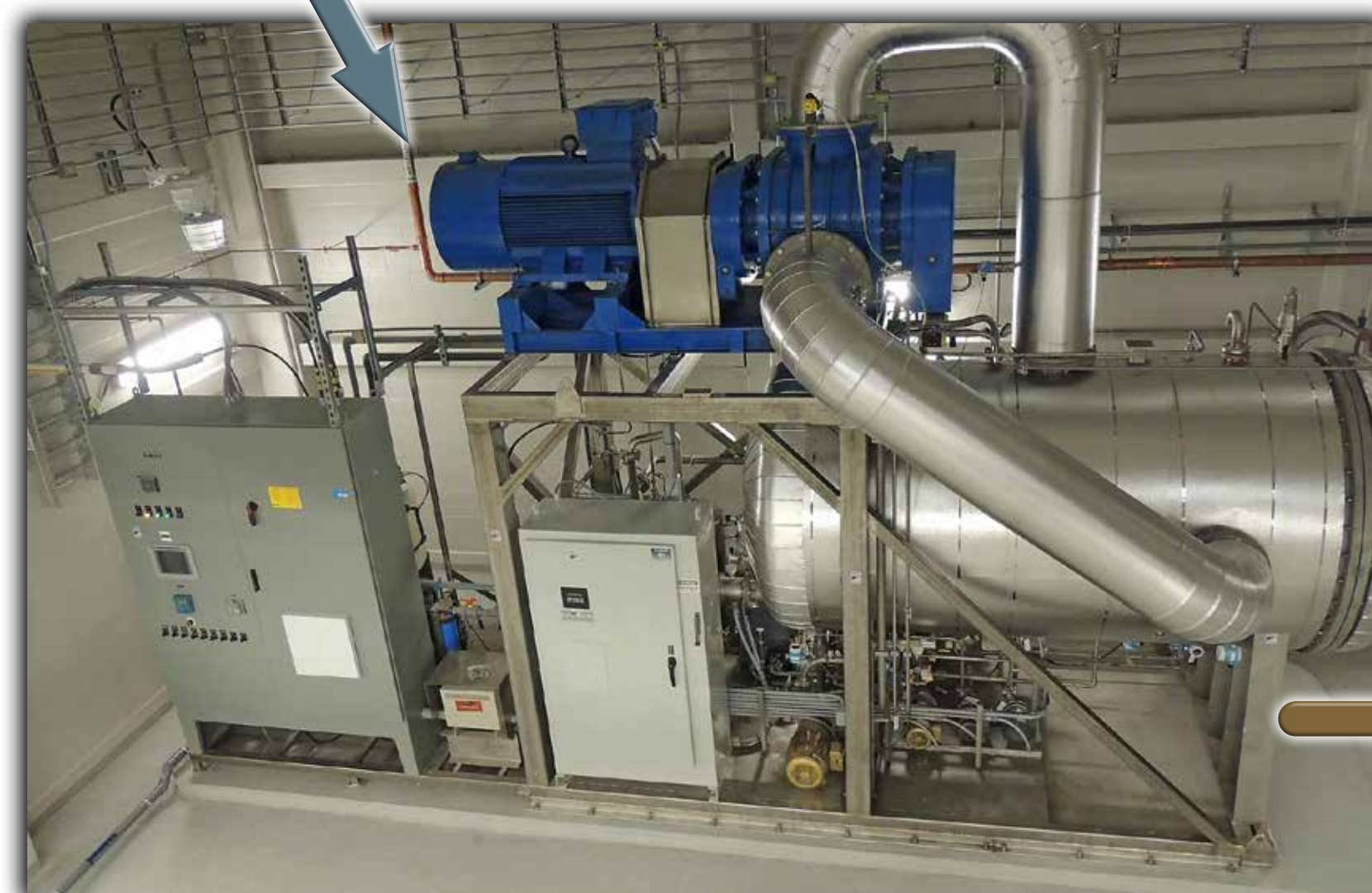
Evaporator Remaining liquid from the clarifier is fed into an evaporator and passes across a heat source. The heat converts the water from liquid to vapour that is recycled back into the treatment process. The remaining watery mixture of insoluble matter is called slurry.
