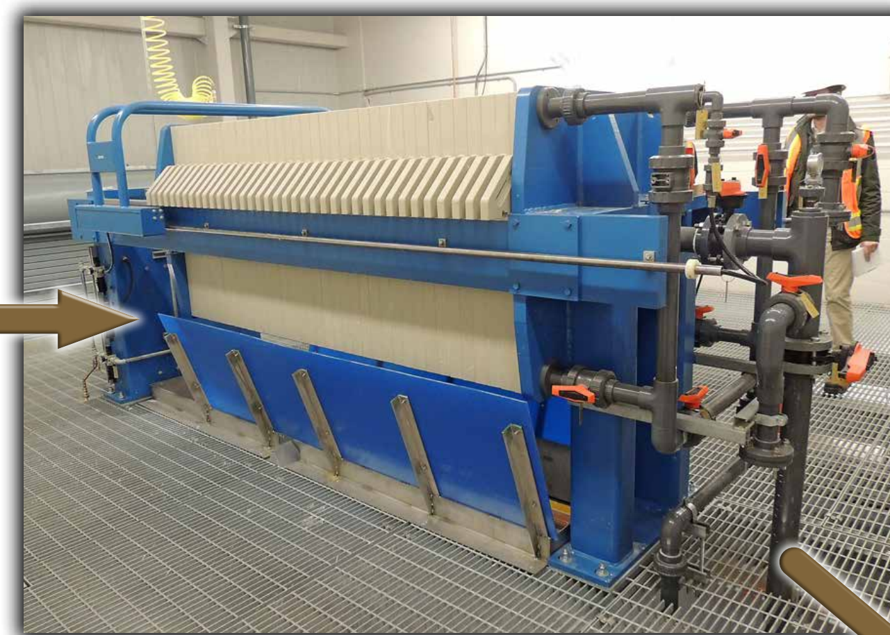
Filter Press Sludge is filtered under mechanical pressure in filtration chambers. The sludge gradually accumulates in the chambers until filter cake is formed. The final compacted filter cake is discharged into collection bins for placement in the mound.
