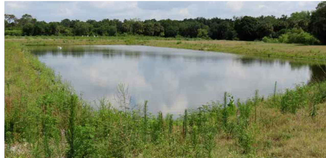
Long-term waste management facility collection pond
