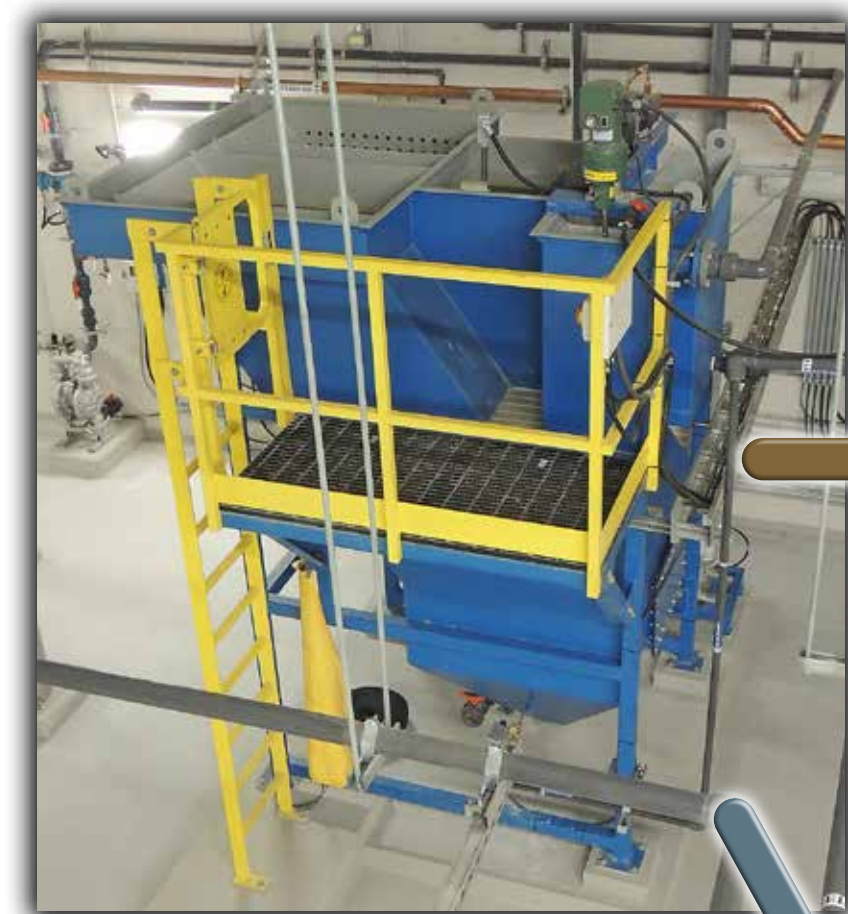
Clarifier Suspended solids from the reverse osmosis system are removed from the liquid and sent to the sludge thickening tank. The remaining liquid is sent to the evaporator.
