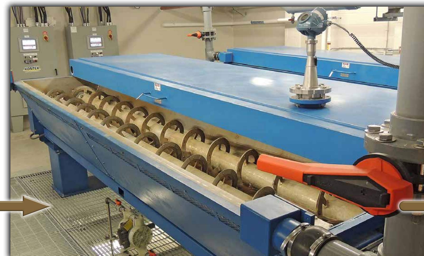
Slurry Dryer Slurry is fed to dryers, where it is dried through a boiling process. The dried product is discharged into specially designed tote bags (right) for placement in the mound. Vapour generated passes through a scrubber before being vented into the atmosphere.
