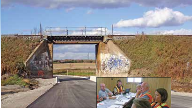
Paving at Elliott Road at CP Rail underpass
