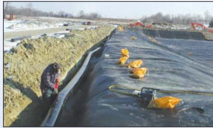
Base liner construction
