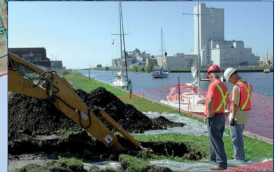
LLRWMO harbour wall soil investigations
