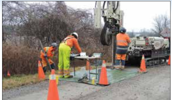
Borehole drilling along the route of the abandoned pipeline
