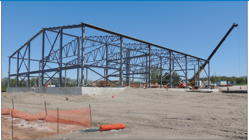
Structural steel erected at new waste water treatment plant
