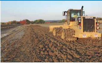
The mound's clay liner is being compacted by machinery known as a "sheep's foot roller."
