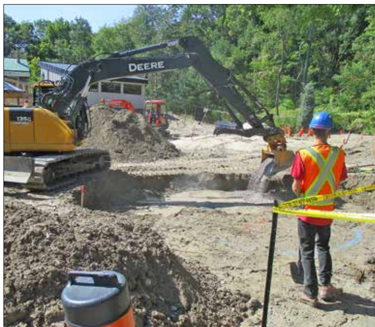
Remove waste, verify soil meets cleanup criteria, and backfill.
