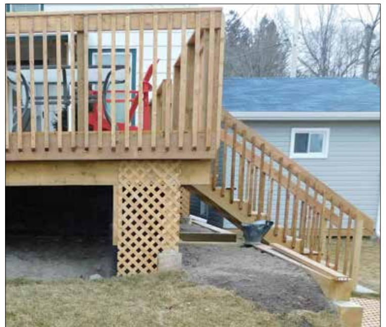
Restore property features including decks, structures, fences and landscaping to building code specifications.
