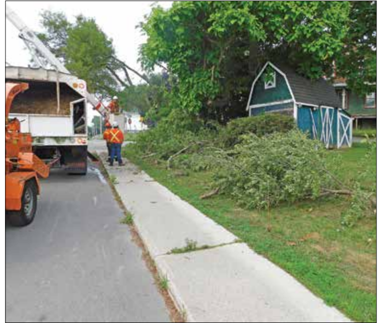
Remove trees, shrubs, impacted structures, store property owner items to facilitate cleanup.
